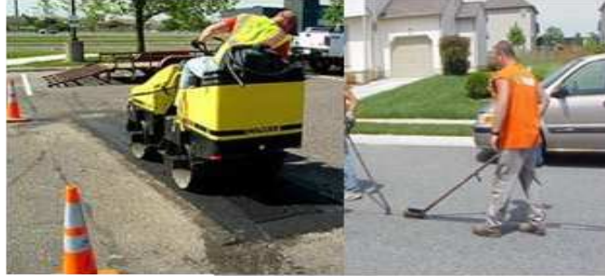
Patching/Crack Sealing
